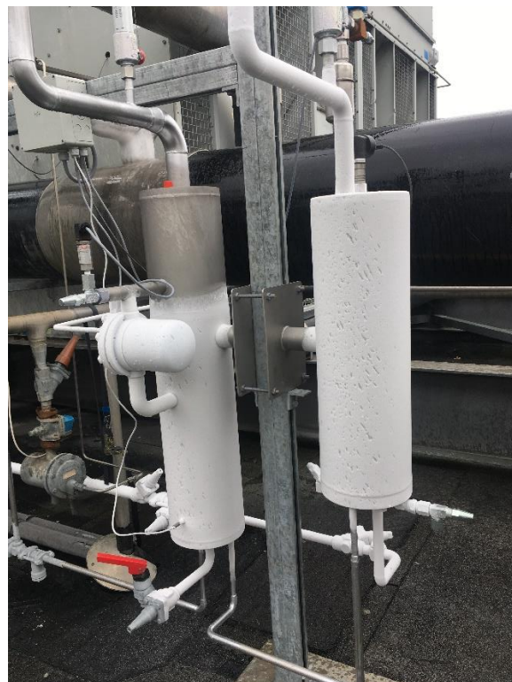
CPAW12 system is back in operation after draining.
