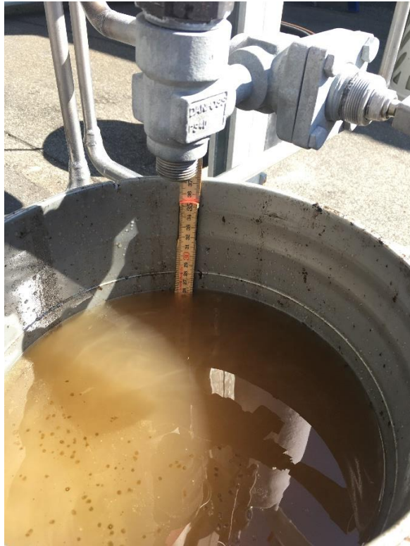
Water and sludge are drained from CPW12
